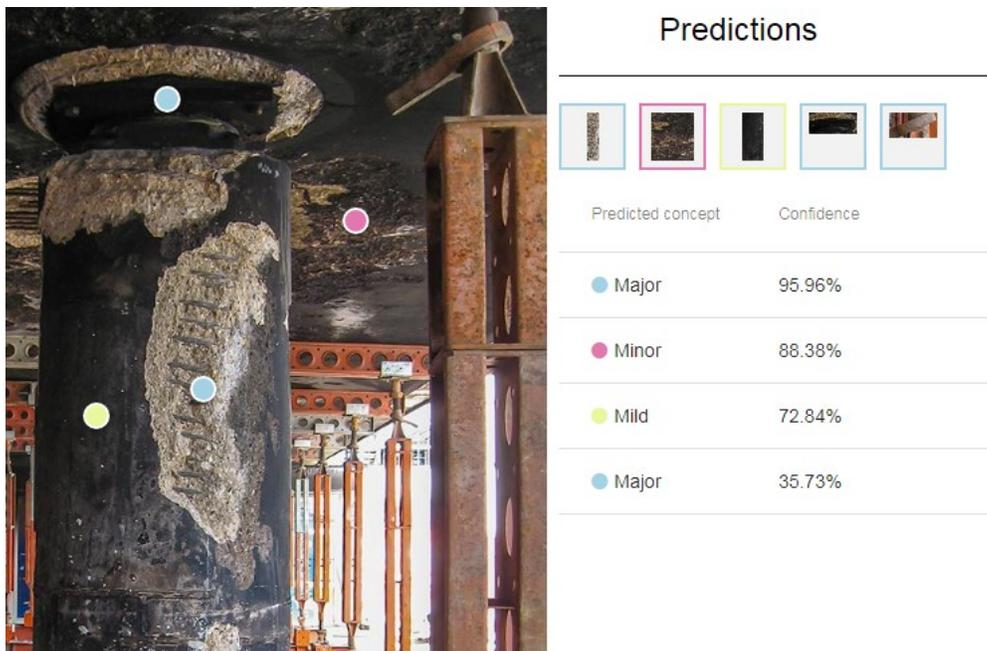
(a) Detecting of spalling magnitude post fire incident
